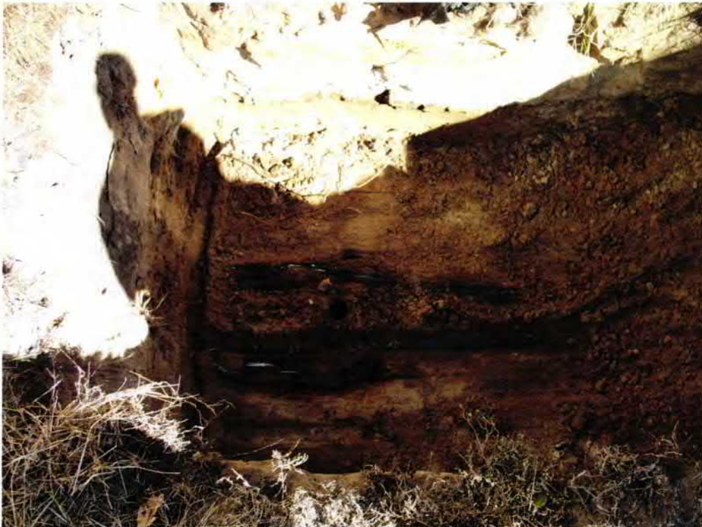
Picture 2: UST 888Cobia excavation in progress.
